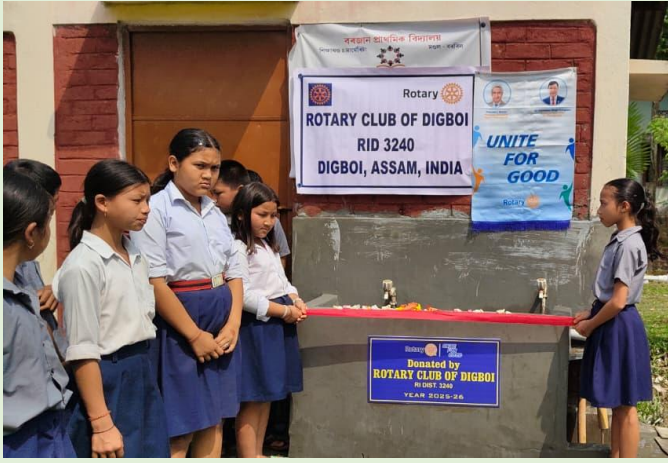
In observance of the March theme of Water, Sanitation and Hygiene (WASH), the Rotary Club of Digboi undertook a meaningful initiative by constructing a concrete wash basin at Borjan LP School.
